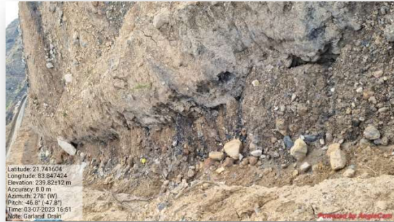
Garland drains provided around the periphery of mine
